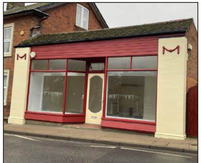
BELOW - THE EX-SHOE SHOP GETTING READY FOR NEW OCCUPANT
